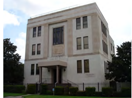
1918 Masonic Lodge Building
