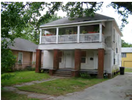
Wilkins House, 1541 Ashland Street
